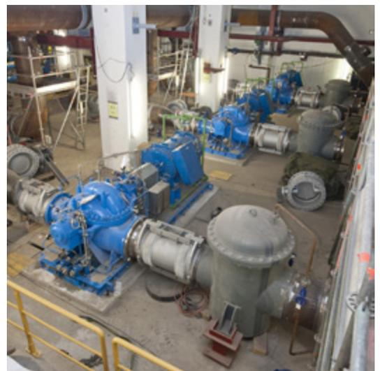
**Figure 7:** Filter type W-SS DN800/PN10 in a newly built power plant in Germany
