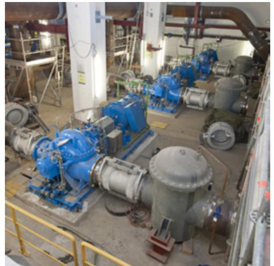
**Figure 7:** Filter type W-SS DN800/PN10 in a newly built power plant in Germany
